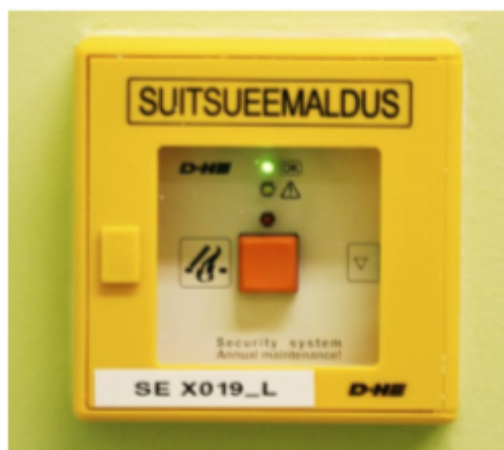
Photo. Smoke vent opening switch.
